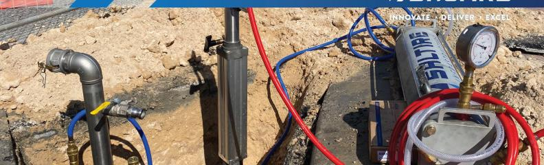
Saltire Infrastructure's technologies focus on water network continuity. Our equipment such as our S-Gate valve system, Live Pipeline Inspection, hot-tapping and line-stopping technology allows us to by-pass the existing network to facilitate repairs and maintenance without disruption.
